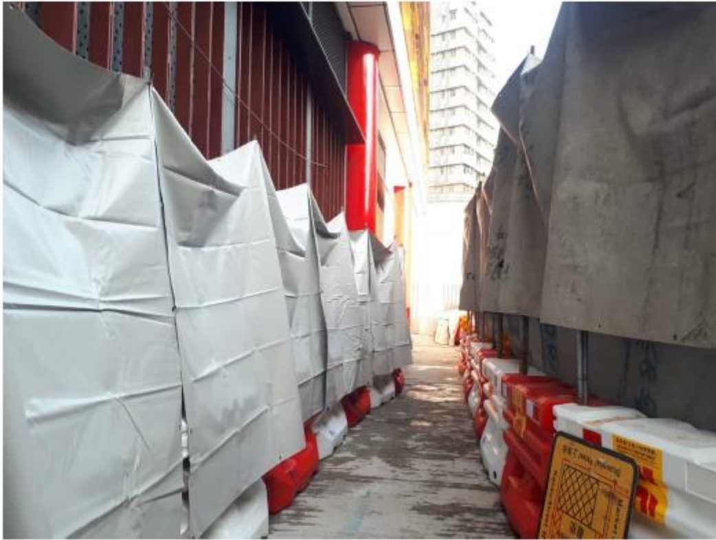
Figure A: The height of two layers of noise barrier mat near the air compressors had been extended
